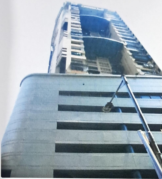
External view of the building
