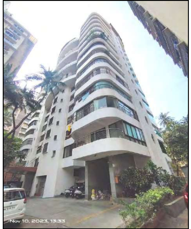
External view of subject property building
