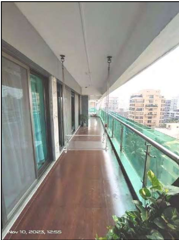
View of balconies attached to subject property
