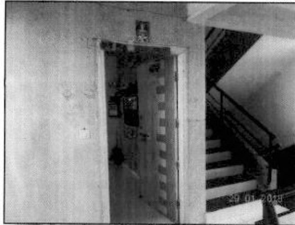
Entrance Door of the Said Asset
