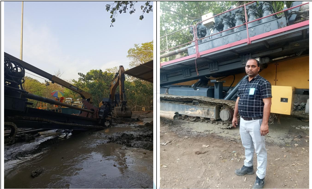
View of Horizontal Directional Drilling, Model- XZ3600
