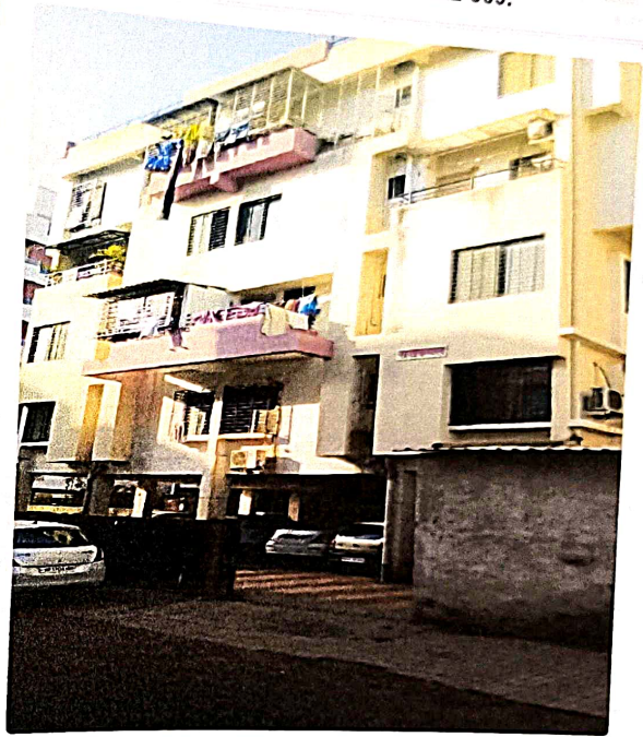
External view of the building
