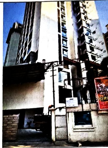
View of Building
