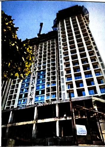
View of Building
