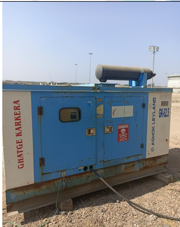
62.5 KVA DG Set, Model.-AL4CTIDG5 at Location-4
