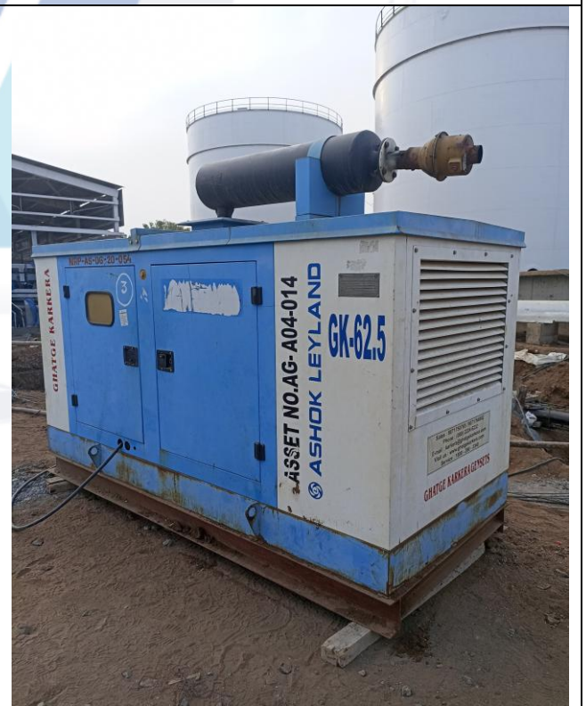
62.5 KVA DG Set, Sr. No.-GRBLR at Location-3
