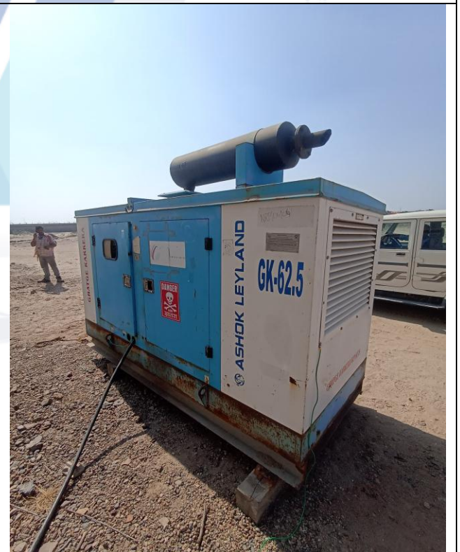
62.5 KVA DG Set, Model.-AL4CTIDG5 at Location-4
