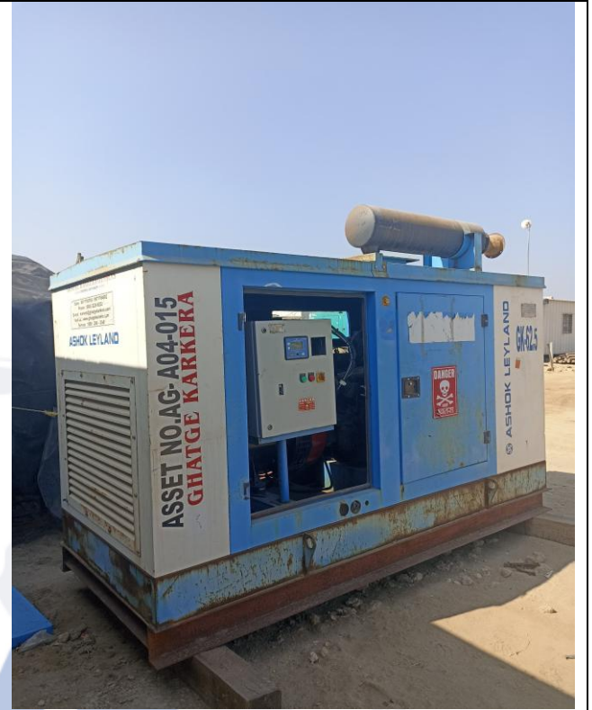
62.5 KVA DG Set, Model.-AL4CTIDG5 at Location-4
