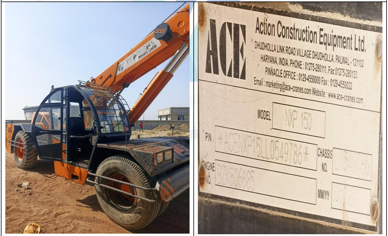
Hydraulic Mobile Crane 15T, Sr. No.-ACENXP15LL0549786 at Location-4
