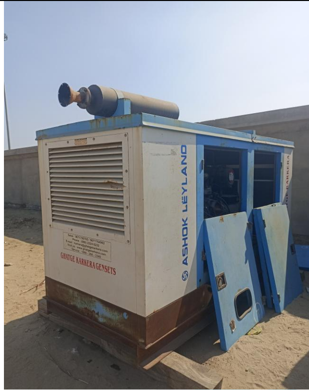
62.5 KVA DG Set, Model.-AL4CTIDG5 at Location-4
