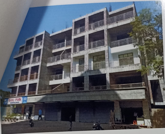
Front view of the building
