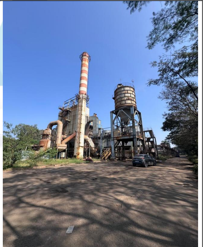
View of Plant
