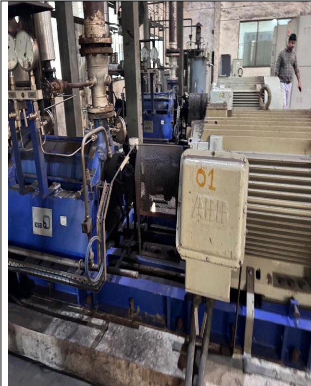
Boiler Feed Pump
