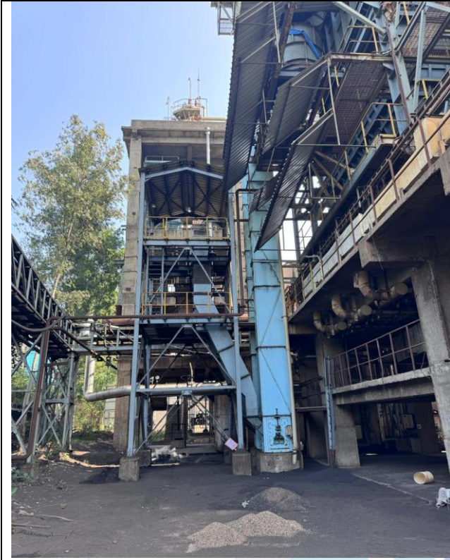
Coal Handling System
