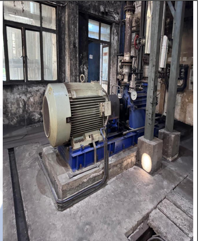
Boiler Feed Pump
