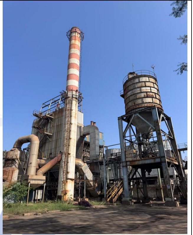
View of Plant
