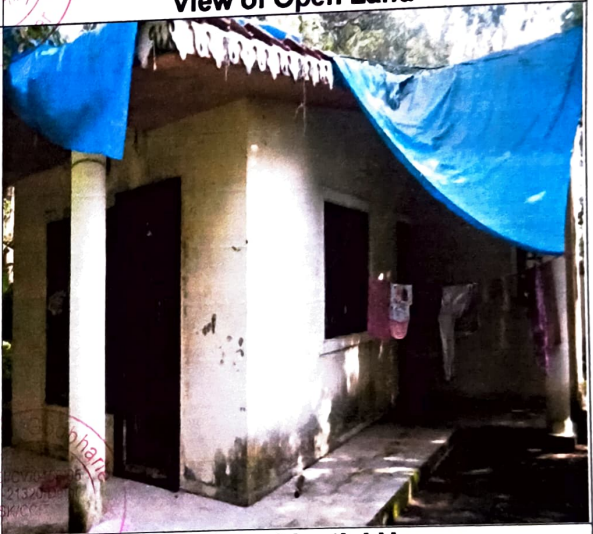
View of Residential House
