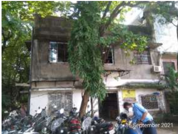
VIEW OF BUILDING
