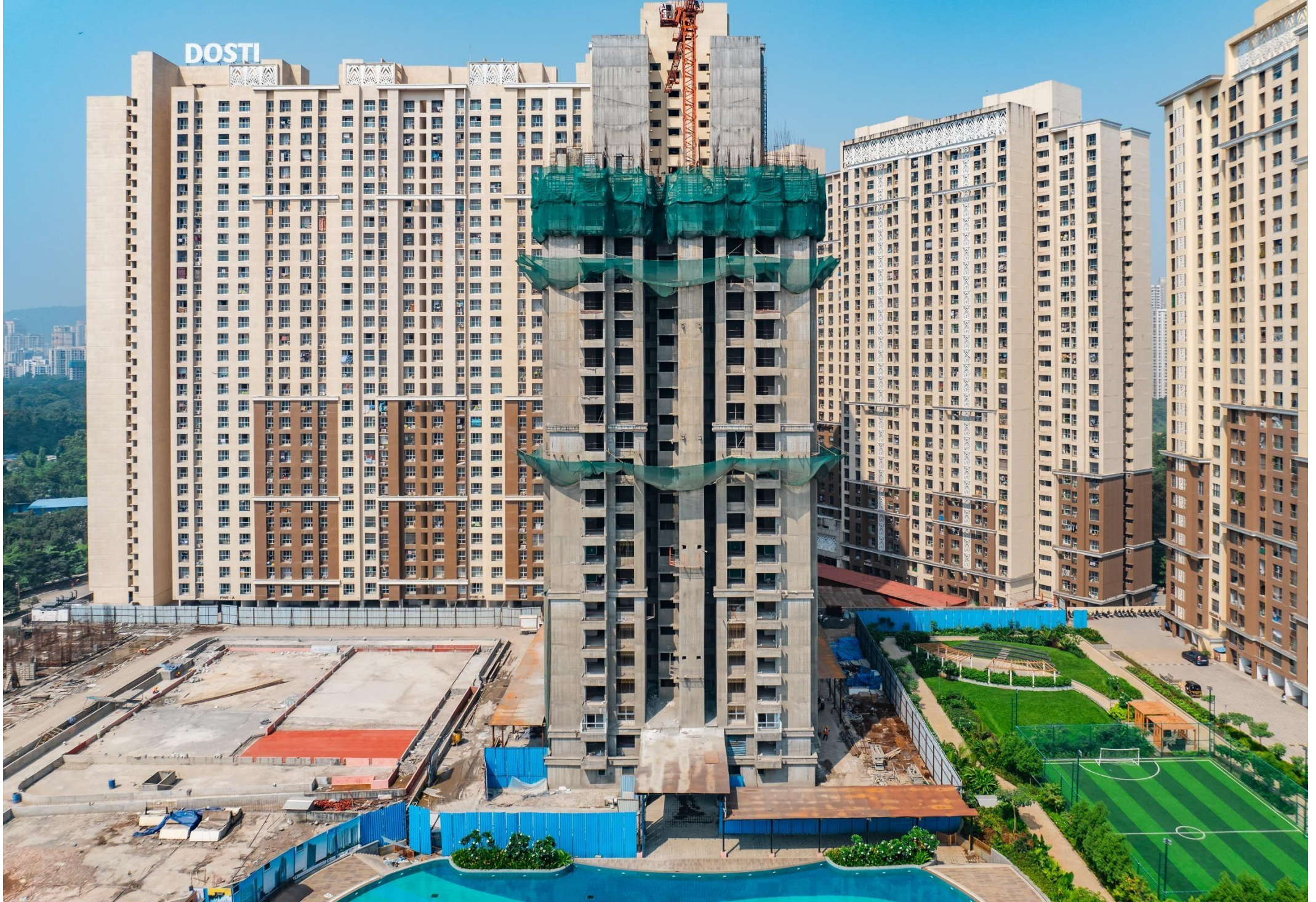
PINE E - 24 TH FLOOR LEVEL SLAB WORK IN PROGRESS
