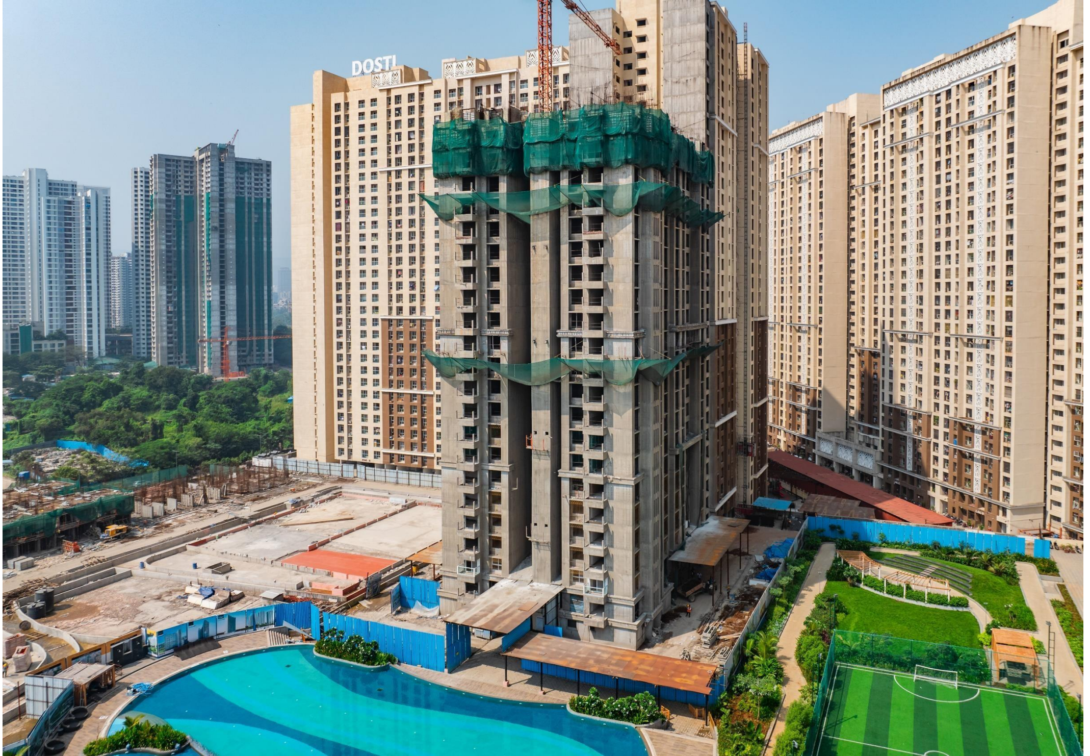
PINE E - 24 TH FLOOR LEVEL SLAB WORK IN PROGRESS
