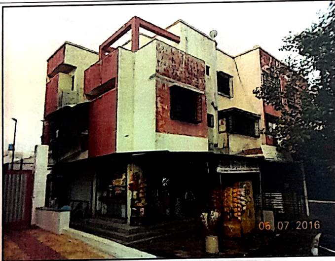
Corner View of the Bldg. - "Bharat" Apt.
