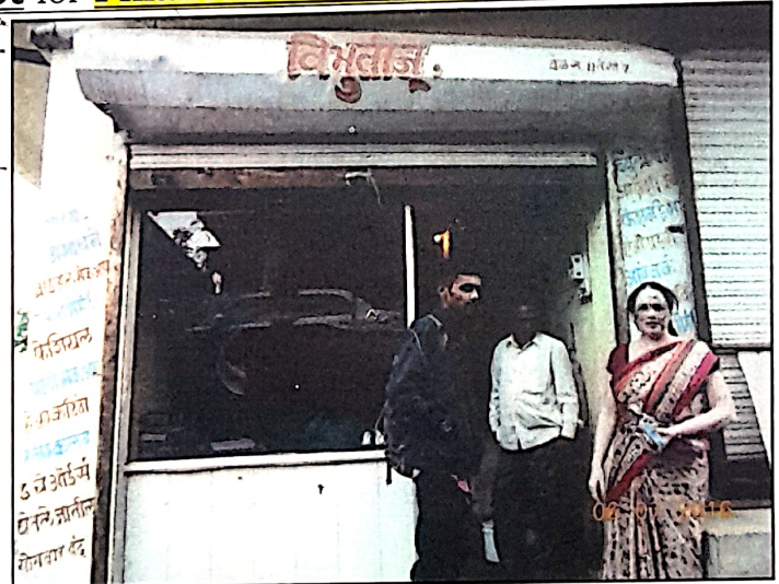
Front View of the Said Asset
