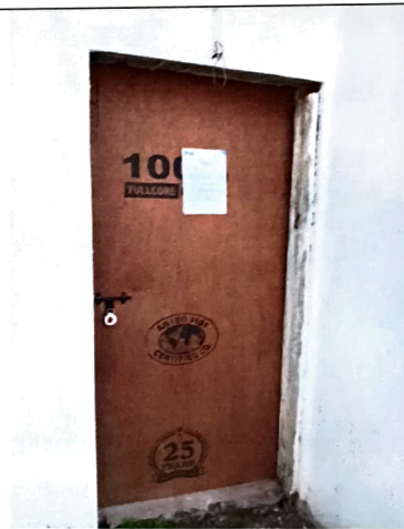
VIEW OF DOOR
