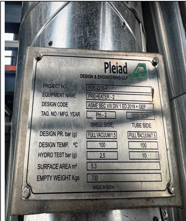
Name Plate of Preheater-2
