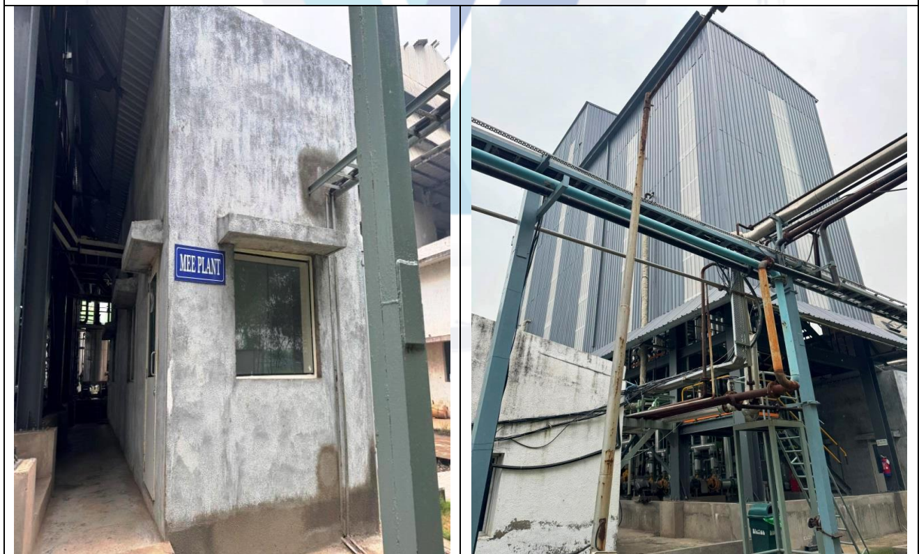
MEE Control Room
