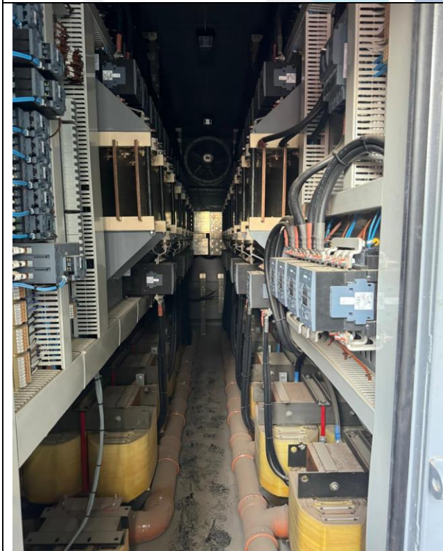
View of 6000 kVA Load Bank, Sr. No. C7110 at Location-1
