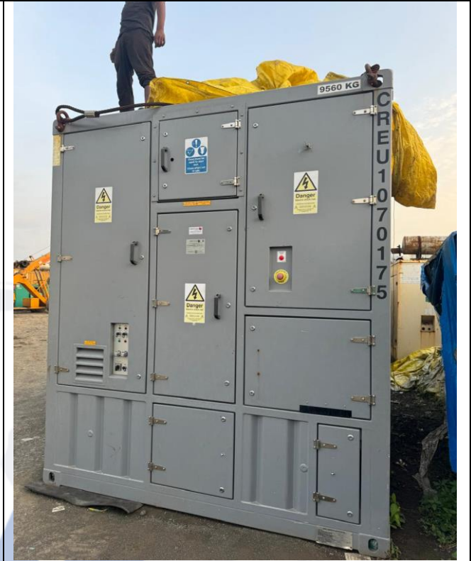
View of 3300 kVA Load Bank, Sr. No. C7017 at Location-3
