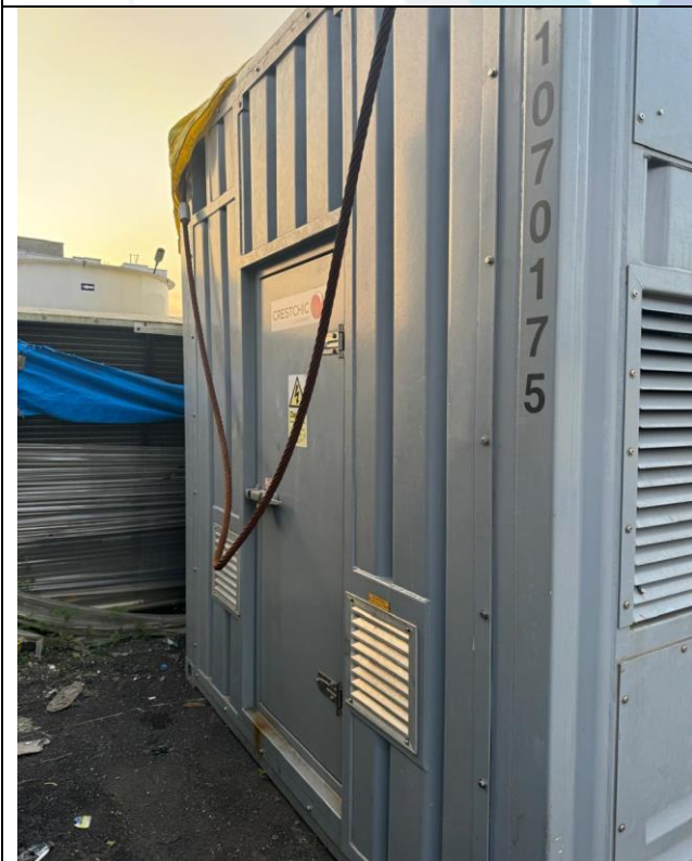
View of 3300 kVA Load Bank, Sr. No. C7017 at Location-3
