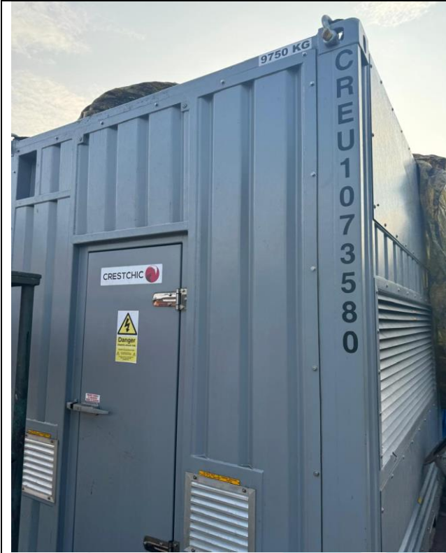
View of 3300 kVA Load Bank, Sr. No. C7358 at Location-2
