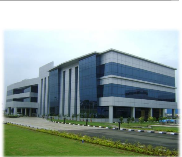
Gold rated LEED Certified Project- M/s. L&T, Hazira, India
