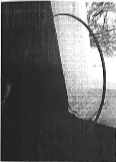
1.A- RC CRACK DEVELOPED IN THE R.C.C. BEAM CORNER.
