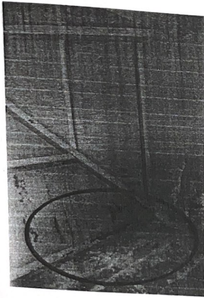
2.B- EXTERNAL SEEPAGE FROM ROOF TOP IS OBSERVED. BUT AT PRESENT FOUND DRY.
