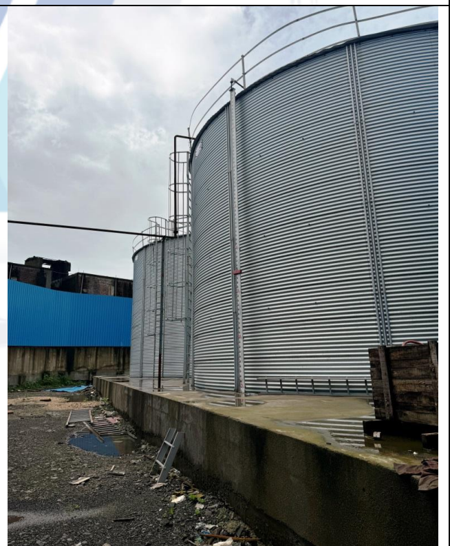
Fire Water Storage Tank
