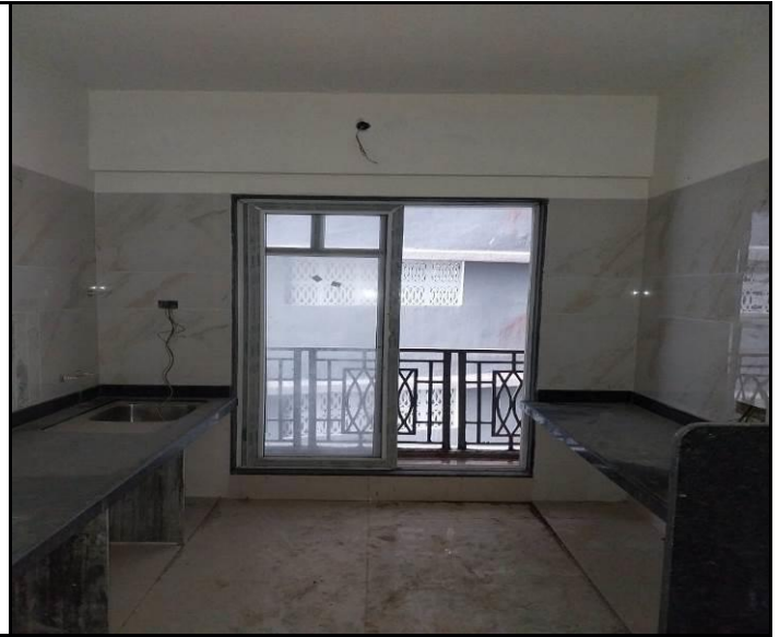
View of kitchen
