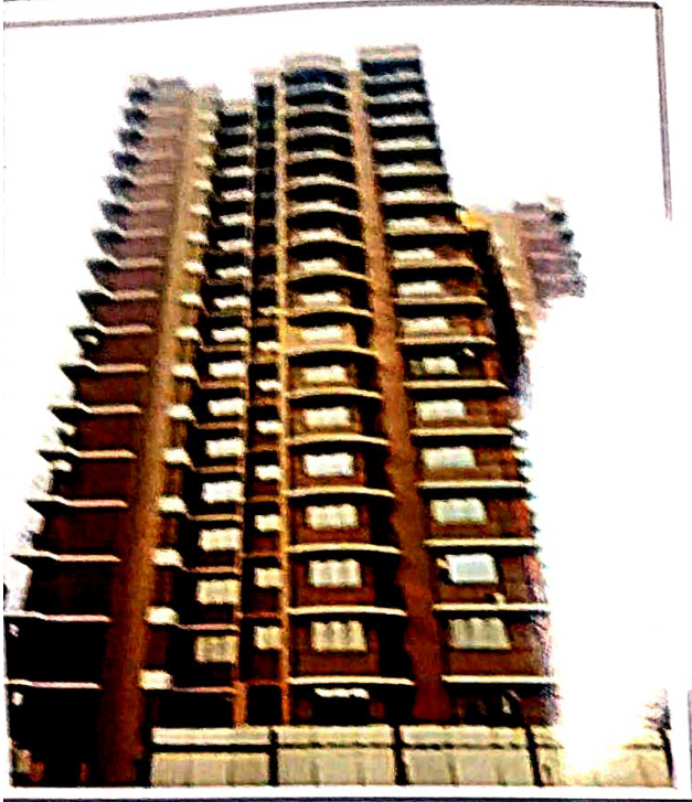
External View of Building
