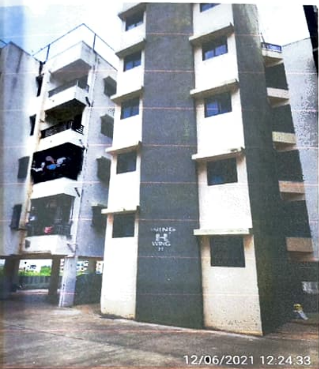
External View Of Building
