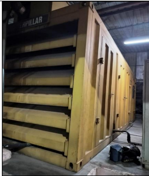
Generator Set, Model-C 18, Capacity-600 KVA, Sr. No. JZB01303 at Location-2
