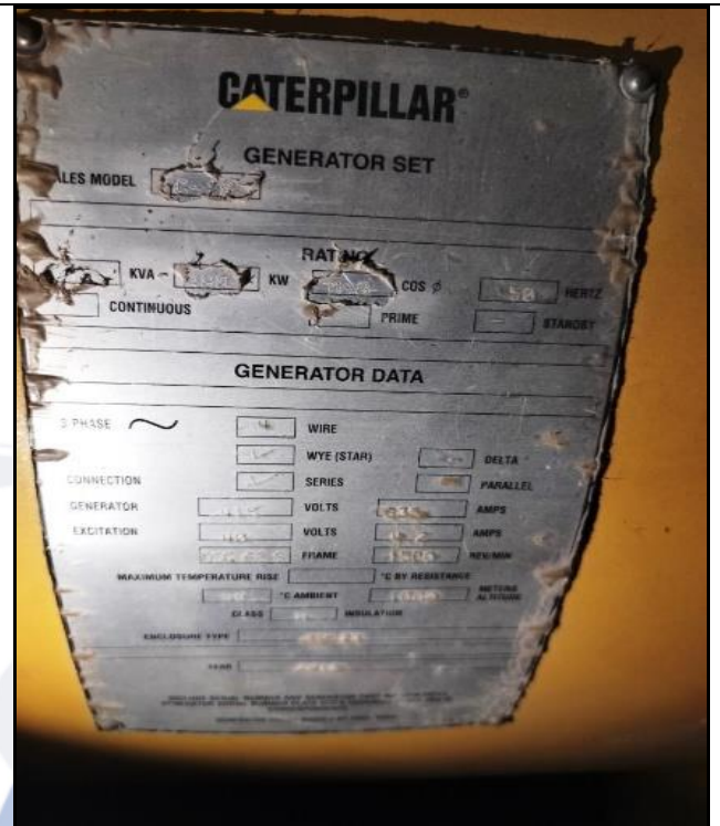
Generator Set, Model-C 18, Capacity-600 KVA, Sr. No. JZB01303 at Location-2
