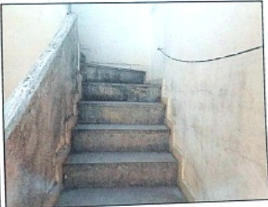
Staircase to Access Roof Terrace
