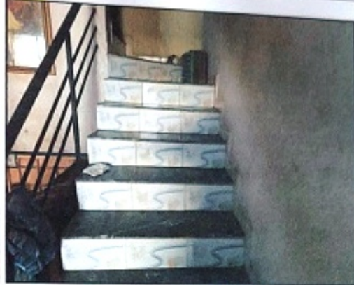
Staircase to access 1 st floor
