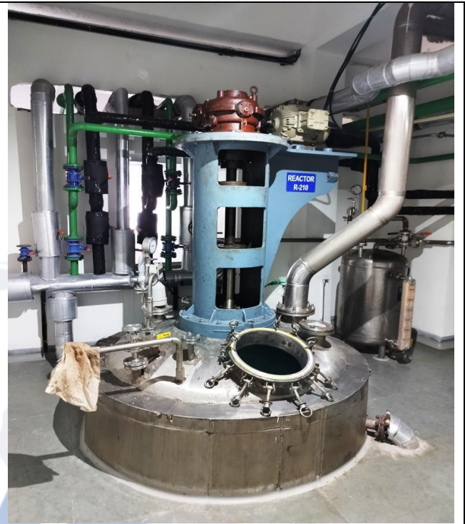
Glass Line Reactor
