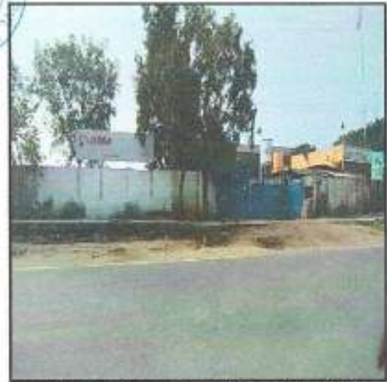
View: Identification of asset- Rear side of factory
