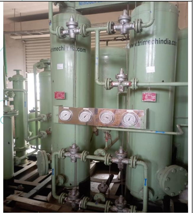
Nitrogen Plant, Capacity 25 m 3 /hr
