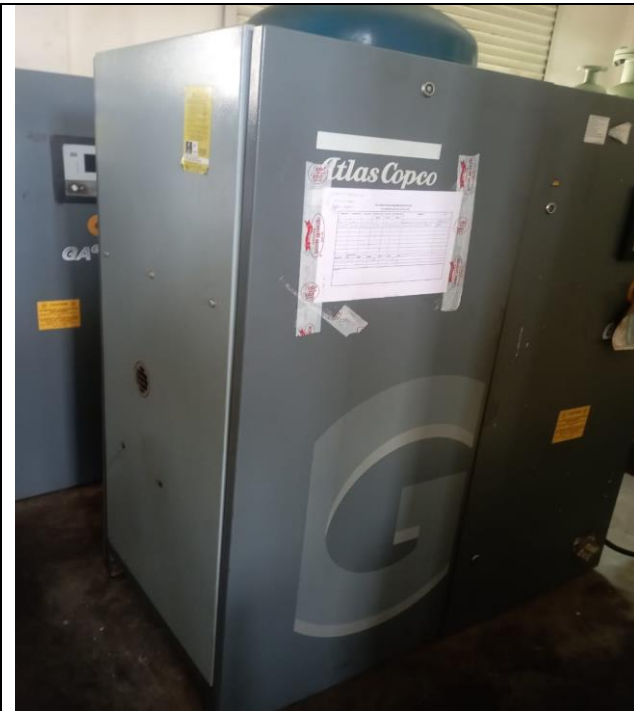
Atlas Copco Make Compressor, Model OGR GAE 17, 7.5 Bar FF with Vertical Air Receiver
