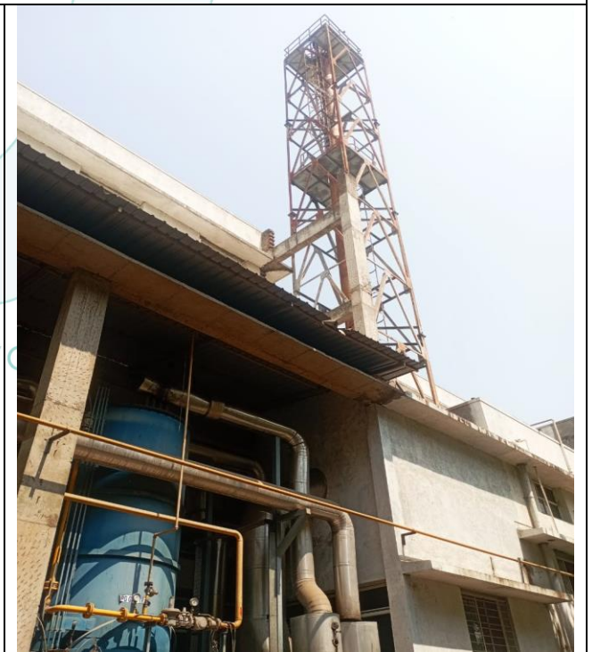
Thermopack Thermic Fluid Heater, Model-TPDI 25/SR No. 11/LDO with Valves
