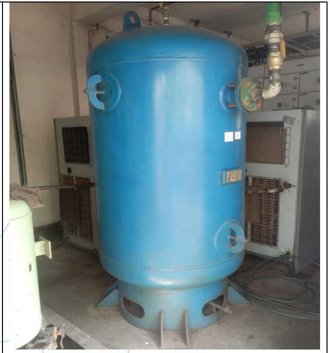
Atlas Copco Make Compressor, Model OGR GAE 17, 7.5 Bar FF with Vertical Air Receiver
