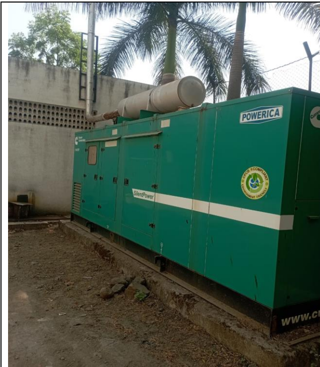
DG Set -400 KVA Cummins, Model No. QSN 14-62
