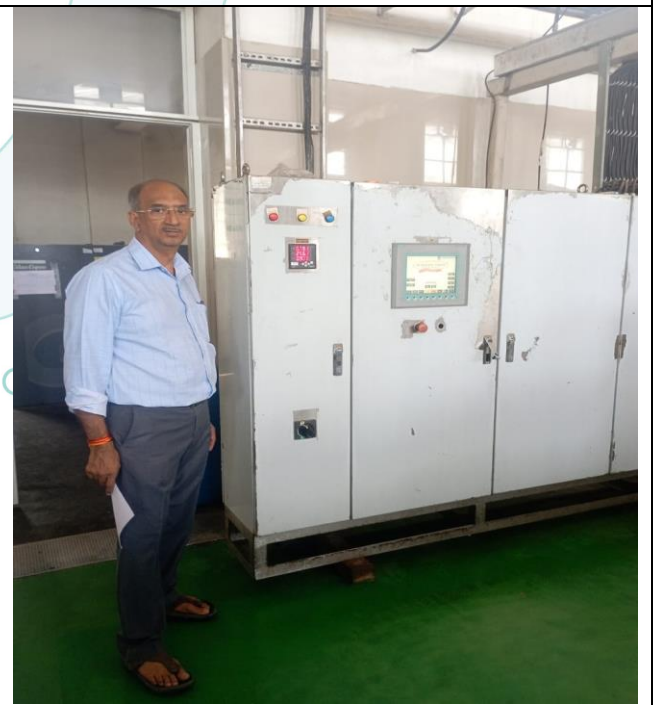
Control Panel with Switchgear (for 750K Wafer Line Project Panel No. 01 & 02
