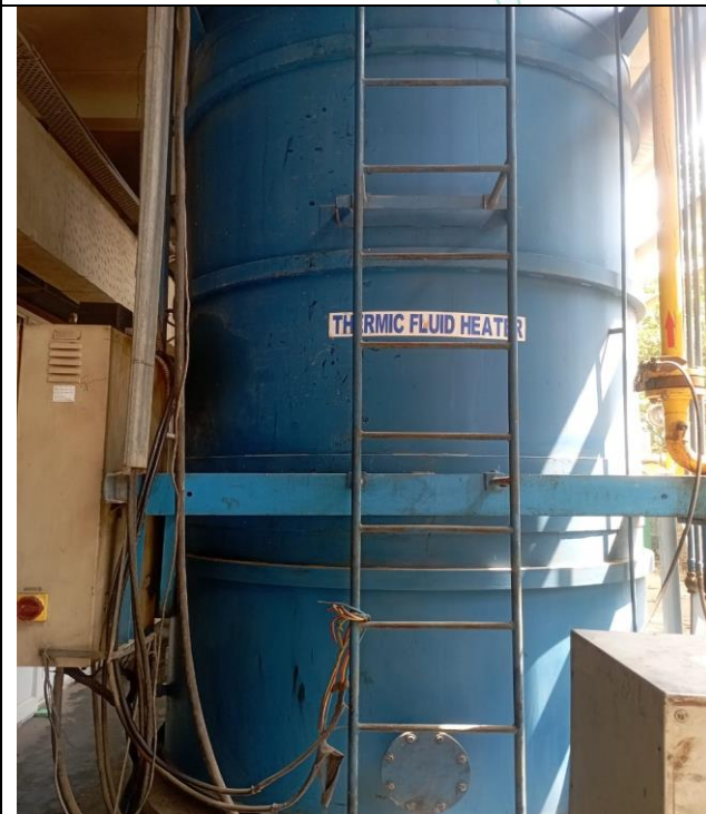
Thermopack Thermic Fluid Heater, Model-TPDI 25/SR No. 11/LDO with Valves
