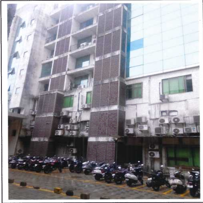
External View of Building
