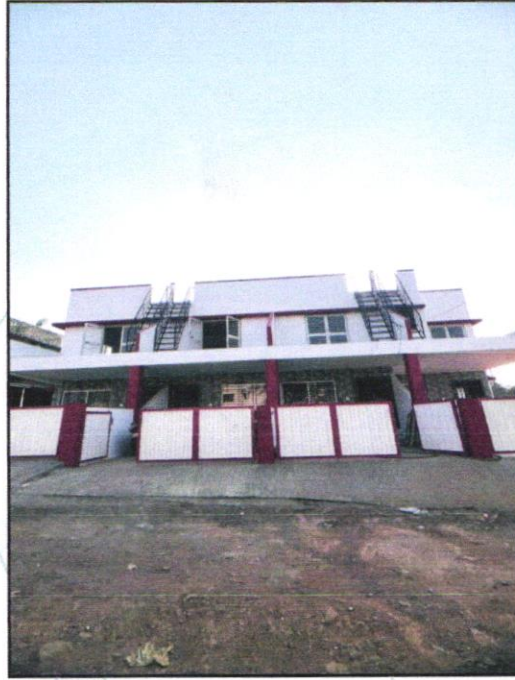
Details of the property under consideration
