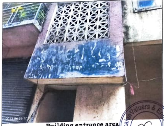
Building entrance area
