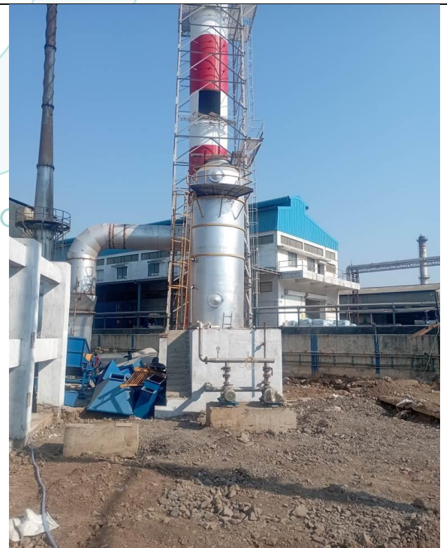
View of Chimney
