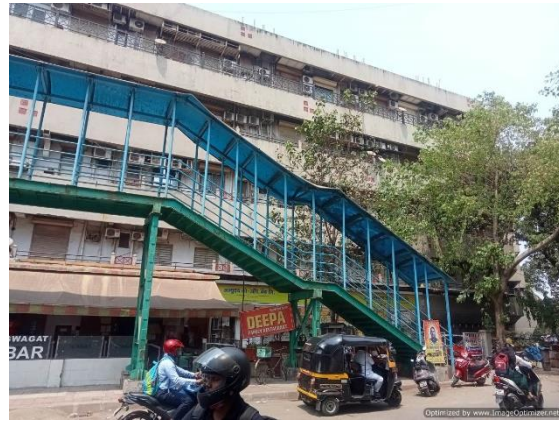
VIEW OF ENTERENCE OF THE BUILDING
