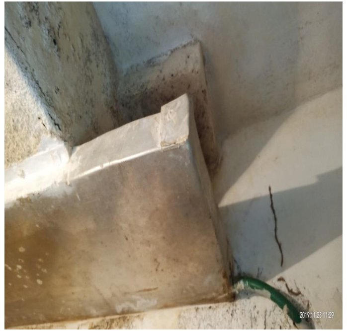
Shop No. 3: Leakage marks on ceiling and try fixed on ceiling for avoid leakage
