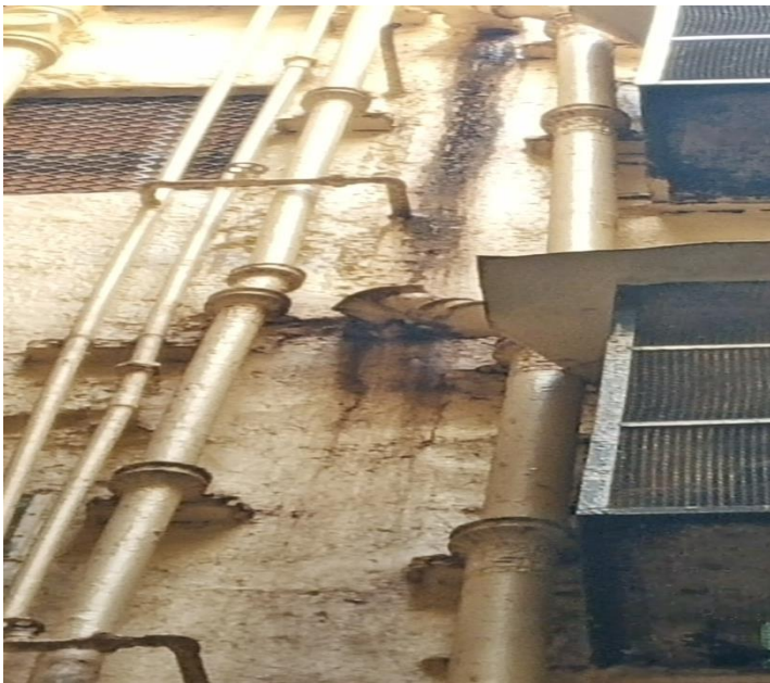
Leakage on Plumbing pipes
