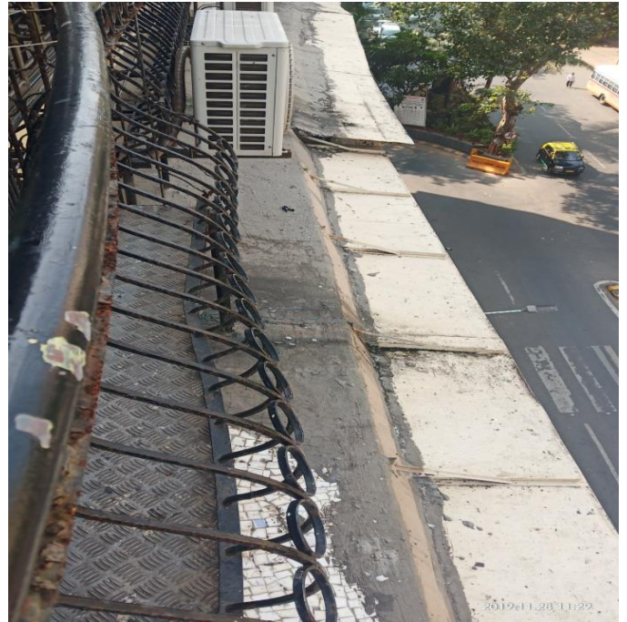
Water proofing coating on 5 th floor level balcony top.
