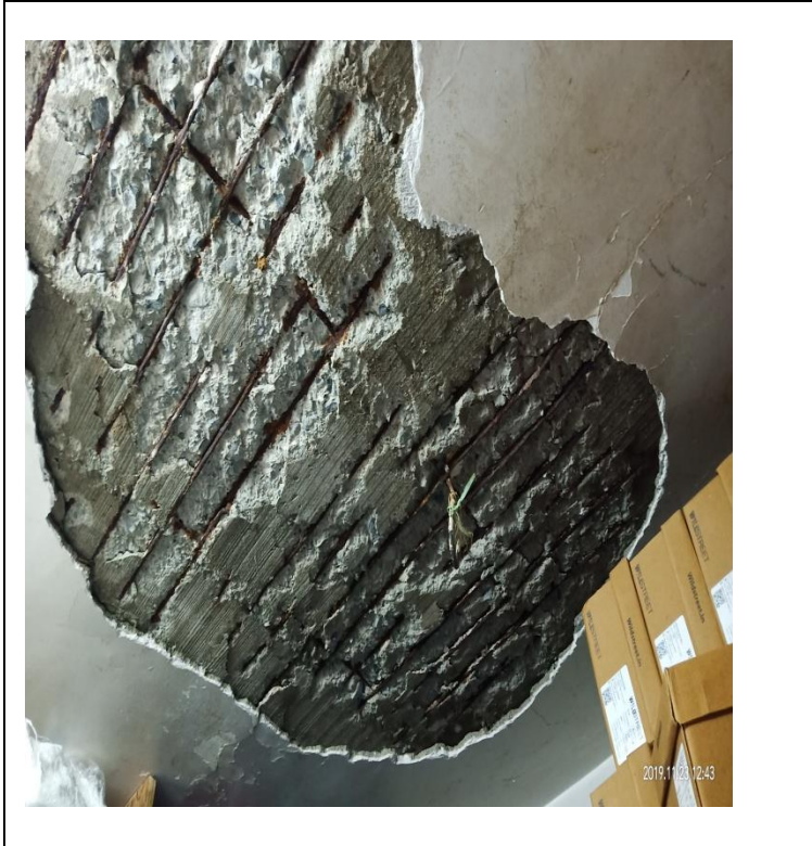
Shop-18: Exposed of reinforcement and heavy corroded on reinforcement .
