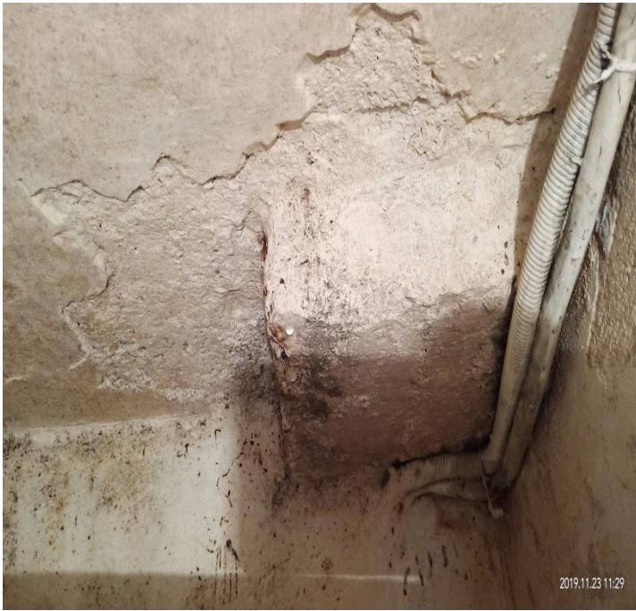
Shop No. 3: Leakage marks on ceiling and try fixed on ceiling for avoid leakage
