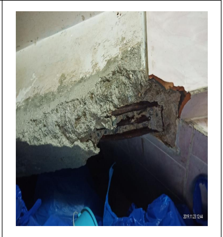
Shop-18: Exposed of reinforcement and heavy corroded on reinforcement .
