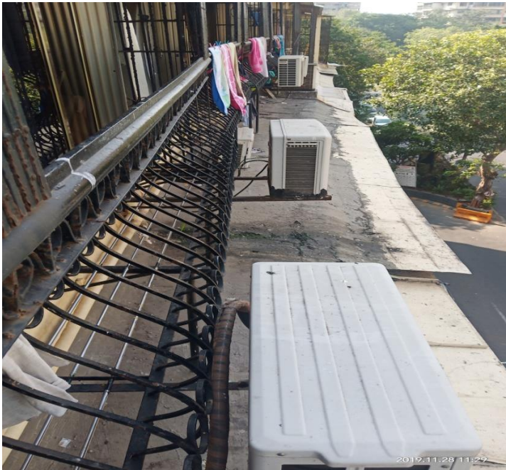
Water proofing coating on 5 th floor level balcony top.
