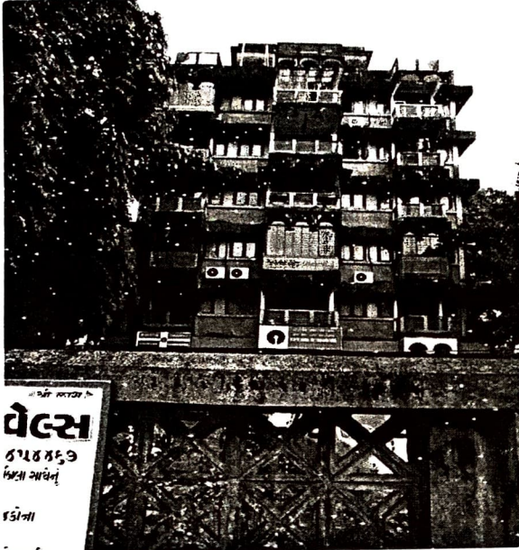
External view of the building
