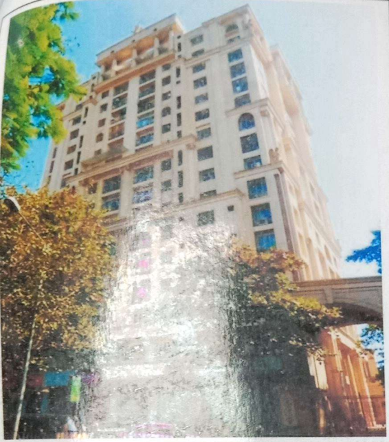
External View of Building
