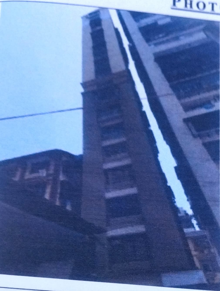
VIEW OF BUILDING
