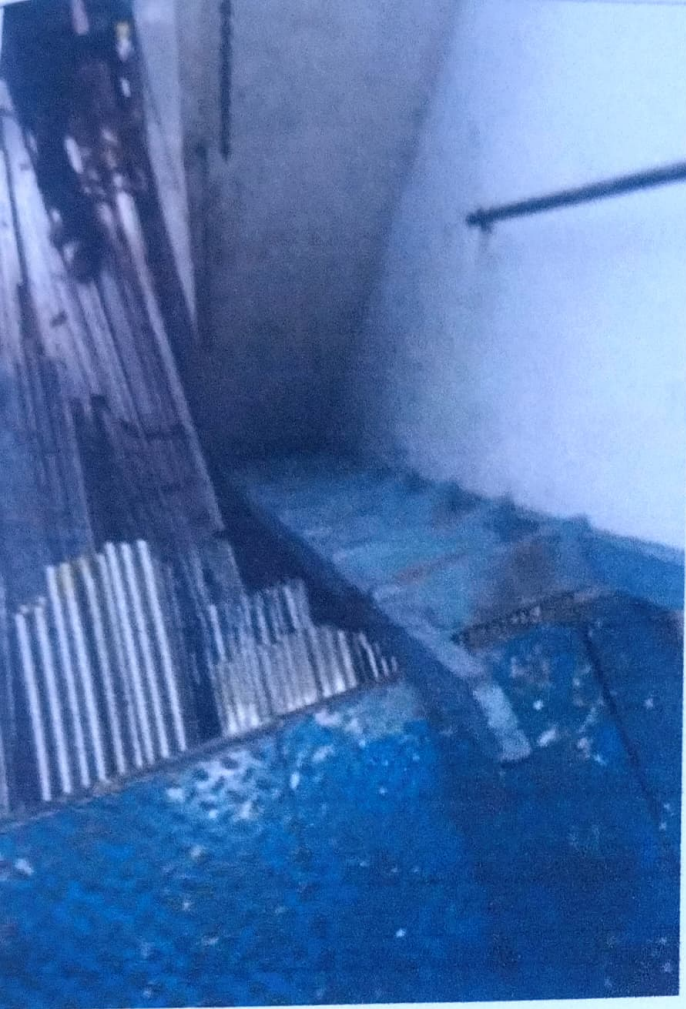
VIEW OF STAIRCASE
