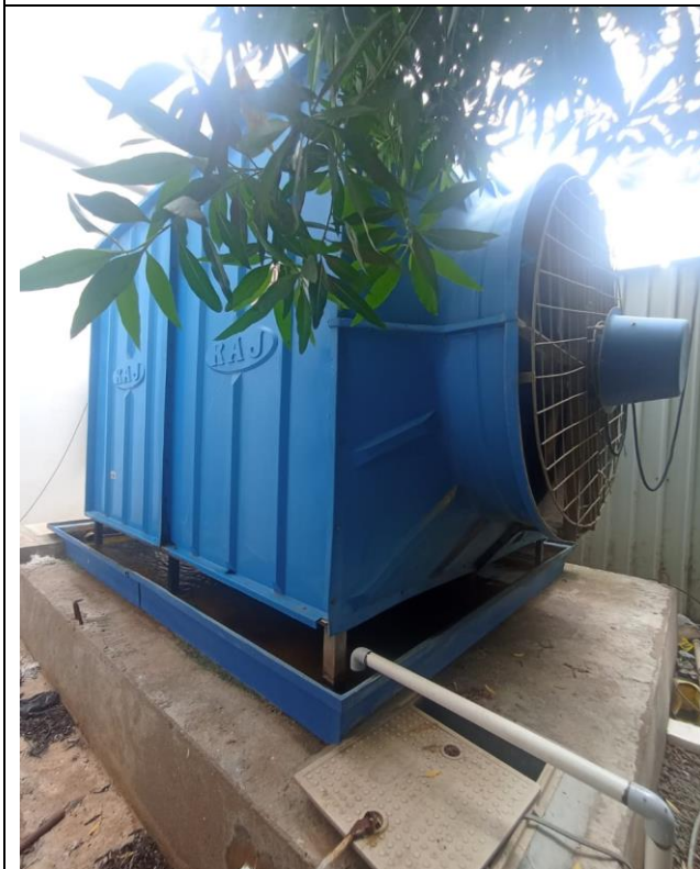
150 TR Cross Flow Cooling Tower with basin, Sr. No. 112179
