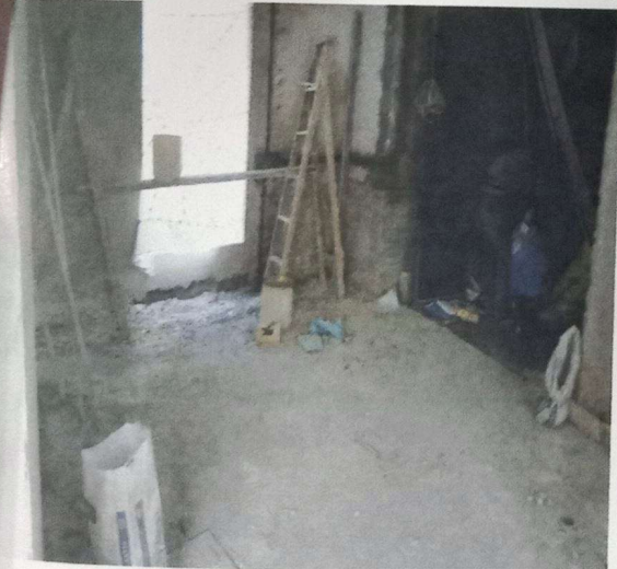
View of the Inside
