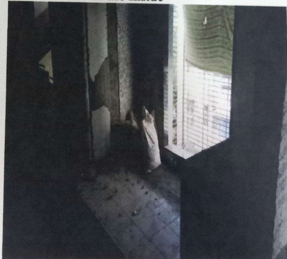
View of the Inside
