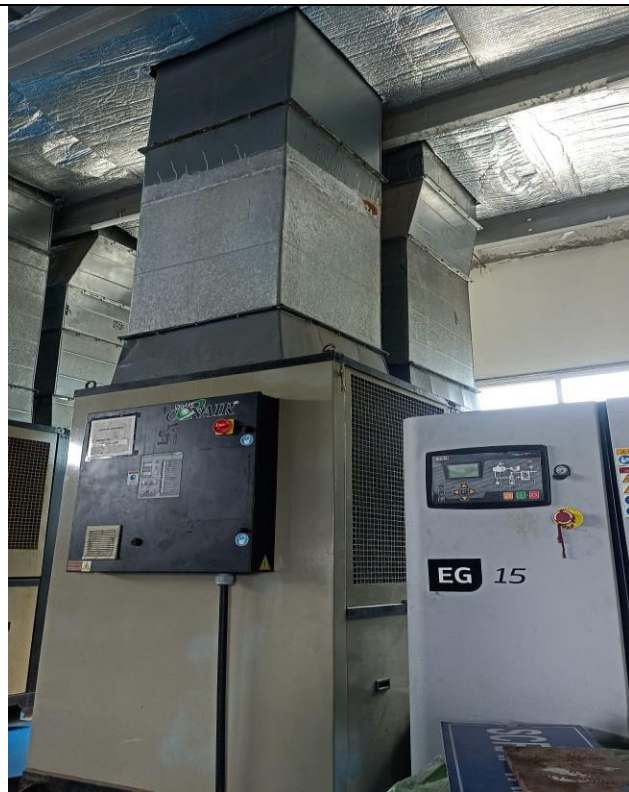
View of Air Cooled Water Chiller EP2A-12 with by pass assembly & Y-Strainer
