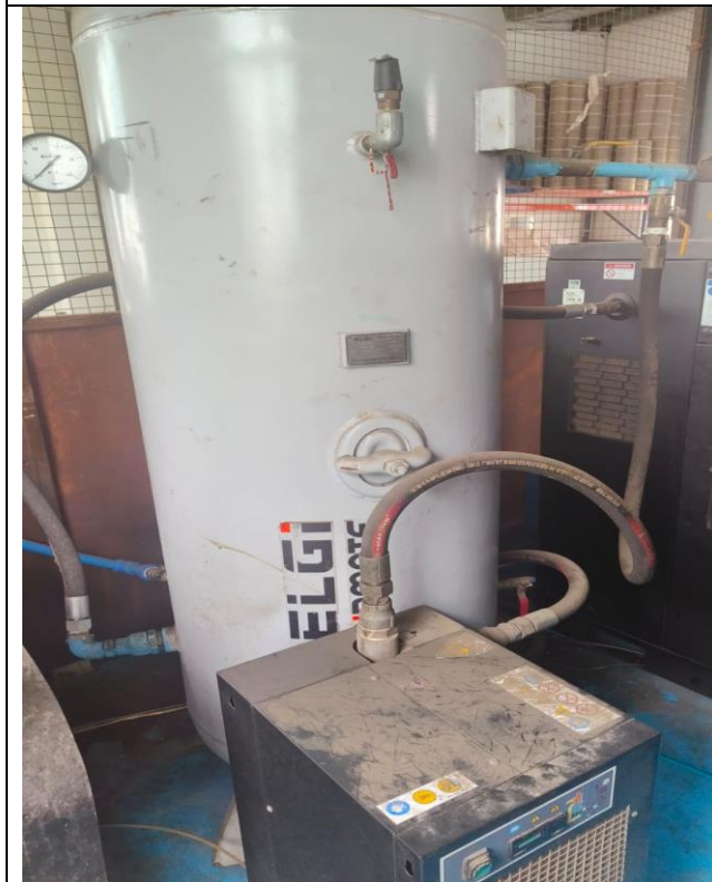
View of Air Receiver VA 00 020 500L 10 ASME 2062V, Fab No.-B19V1541
