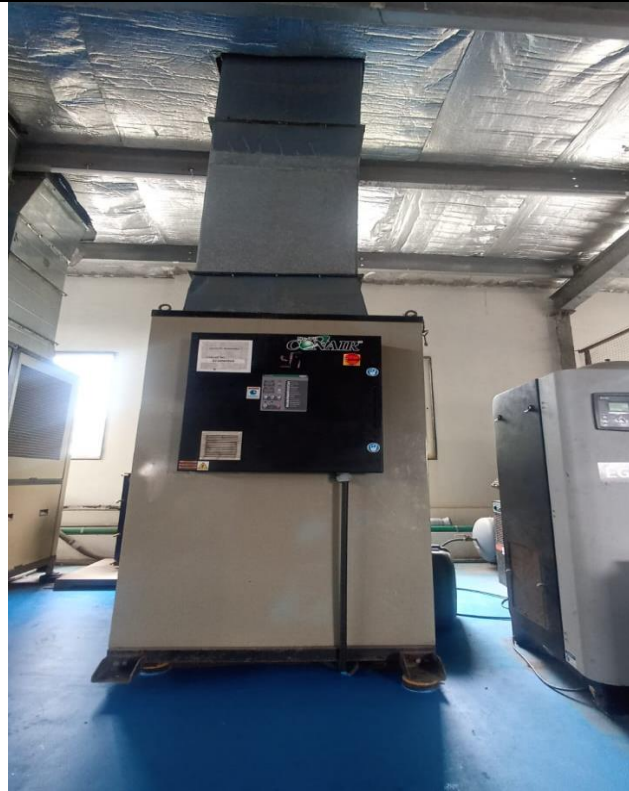
View of Air Cooled Water Chiller EP2A-12 with by pass assembly & Y-Strainer, Sr. No. 3501/07/2019
