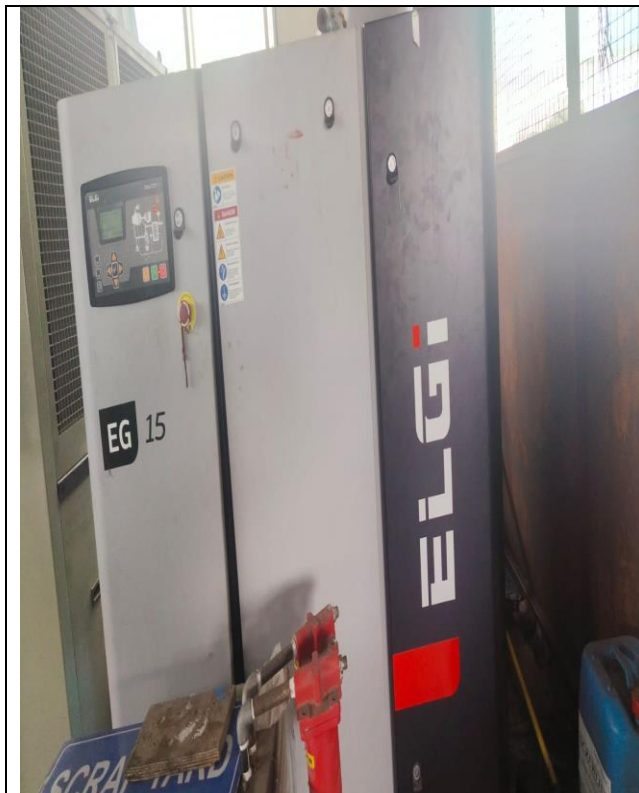
View of EG 15-10 400V/50 Hz Screw Air Compressor, Fab No. BSIS038895
