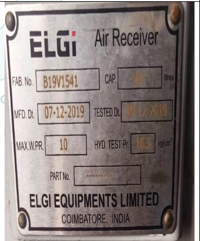
View of Air Receiver VA 00 020 500L 10 ASME 2062V, Fab No.-B19V1541
