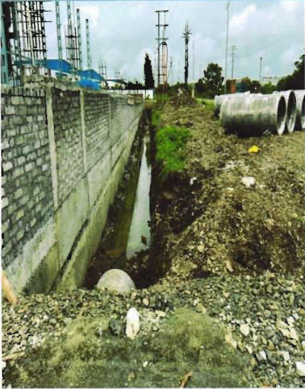
External Storm Water Drain
