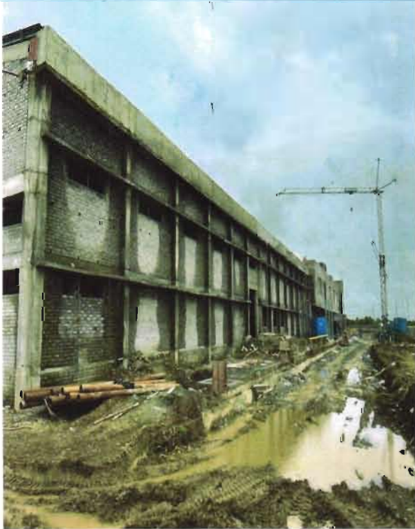
View of Warehouse-1 (Main Plant Building)
