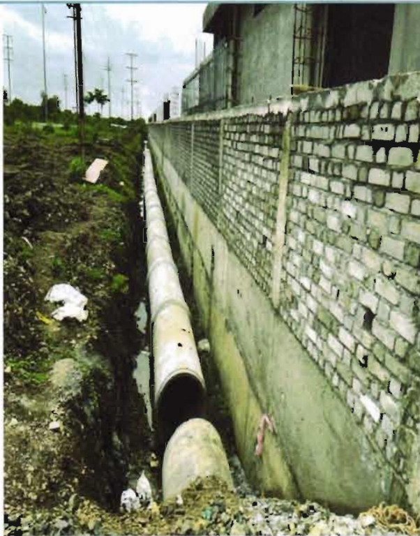
External Storm Water Drain
