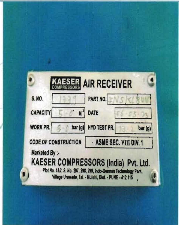
Name Plate of Air Receiver 5 m 3
