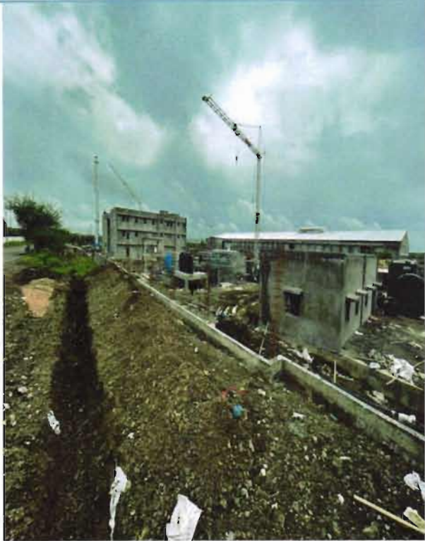
Storm Water Drain
