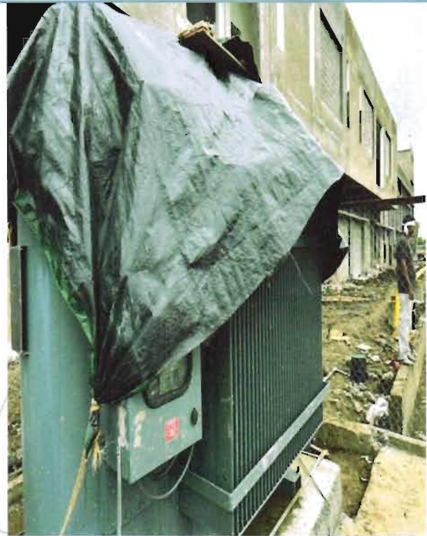
Hermetically Sealed Distribution Transformer-1600 KVA (OLTC Indoor), Sr. No. DI-31803
