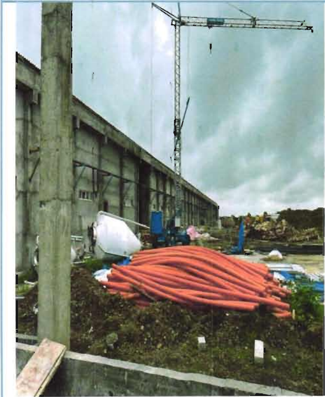
View of Warehouse-1 (Main Plant Building)
