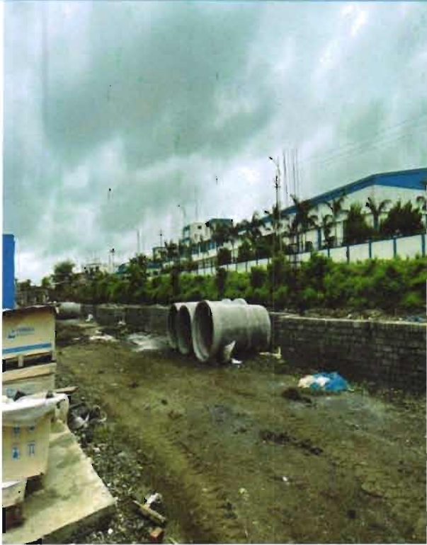
Hume Pipes for Drainage
