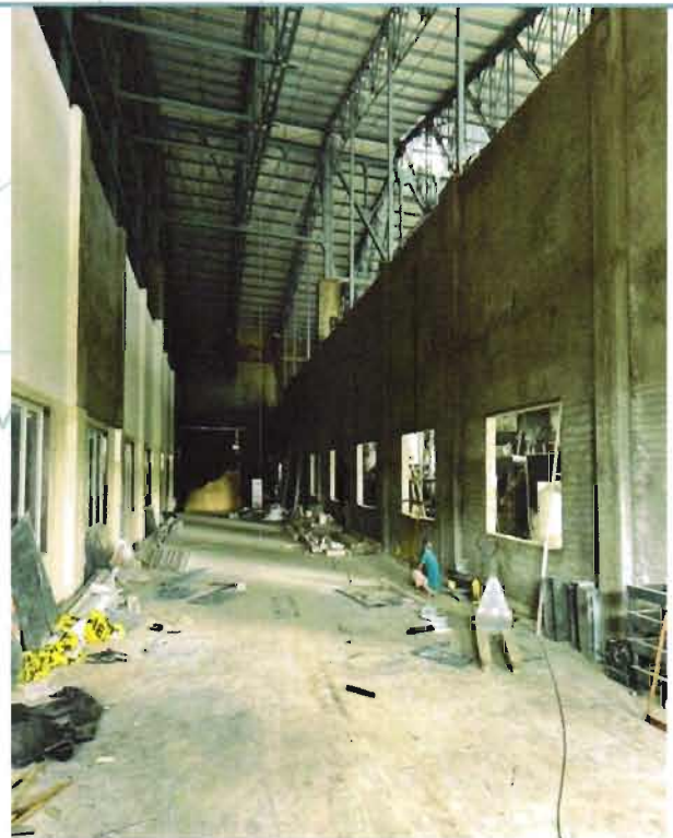
Batch Making Bay
