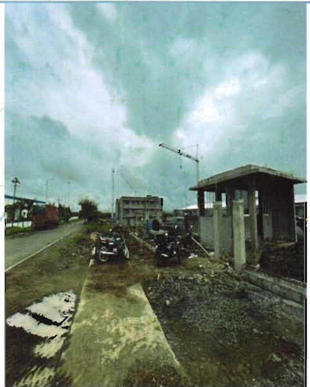
Security Cabin at main Gate
