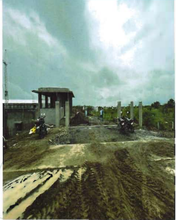
Main Entrance Gate
