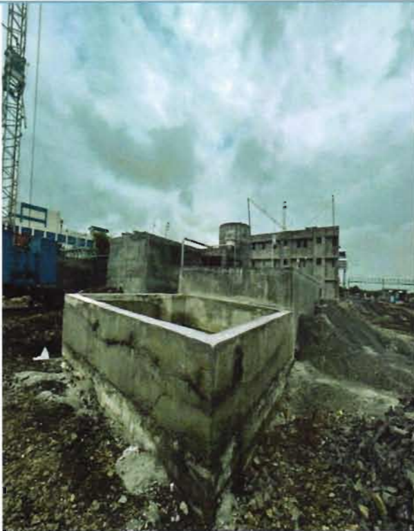
View of ETP
