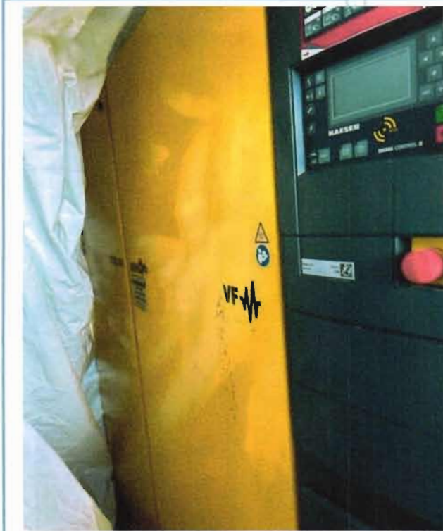
Rotary Screw Compressor
