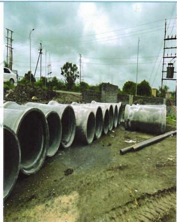
Hume Pipes for Drainage
