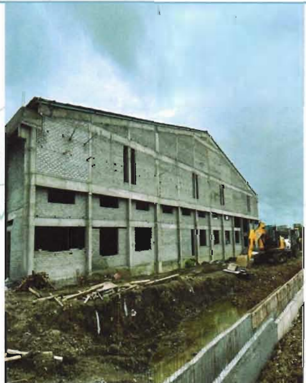
View of Warehouse-1 (Main Plant Building)
