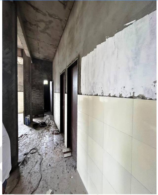
Internal View of Male Quarters
