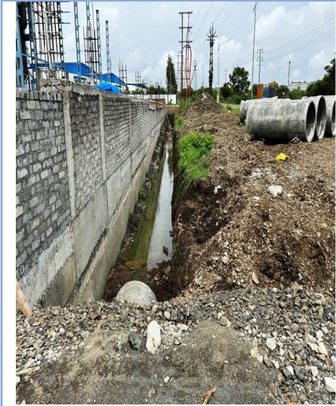
External Storm Water Drain
