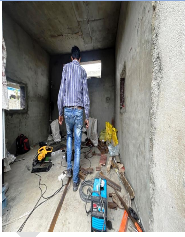
ETP Panel Room
