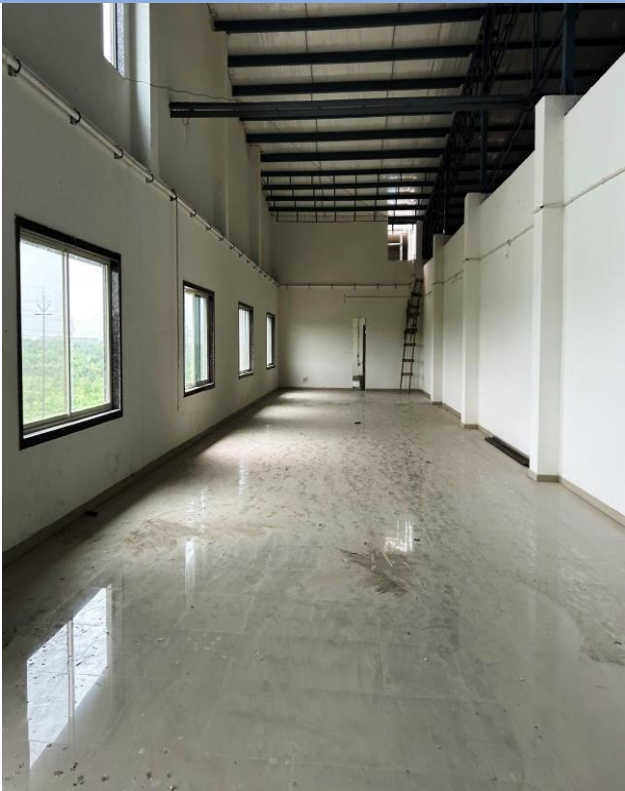
1st Floor Hall and Director Accomodation
