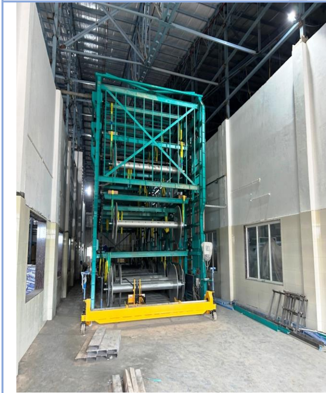
Beam Storage -Stacker
