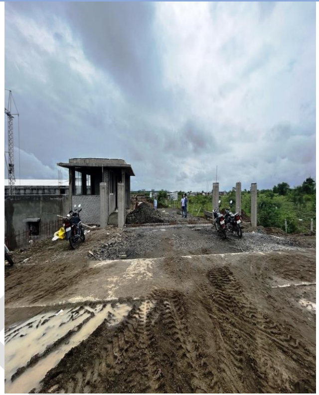
Main Entrance Gate
