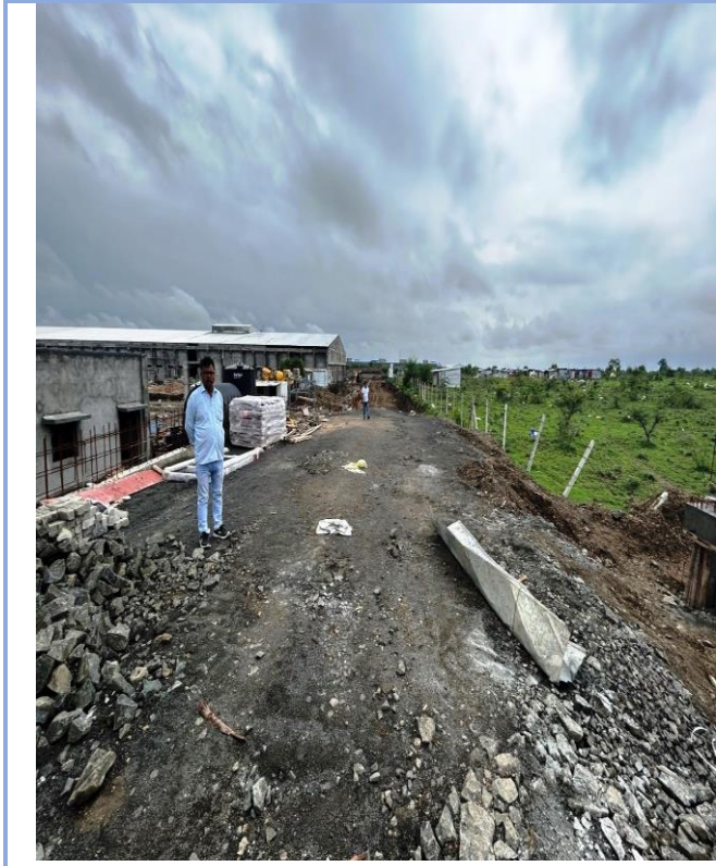
Ramp near main gate
