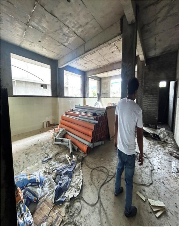
Internal View of Male Quarters
