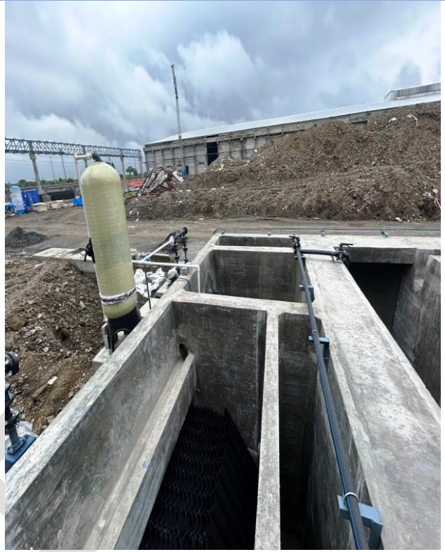
View of STP
