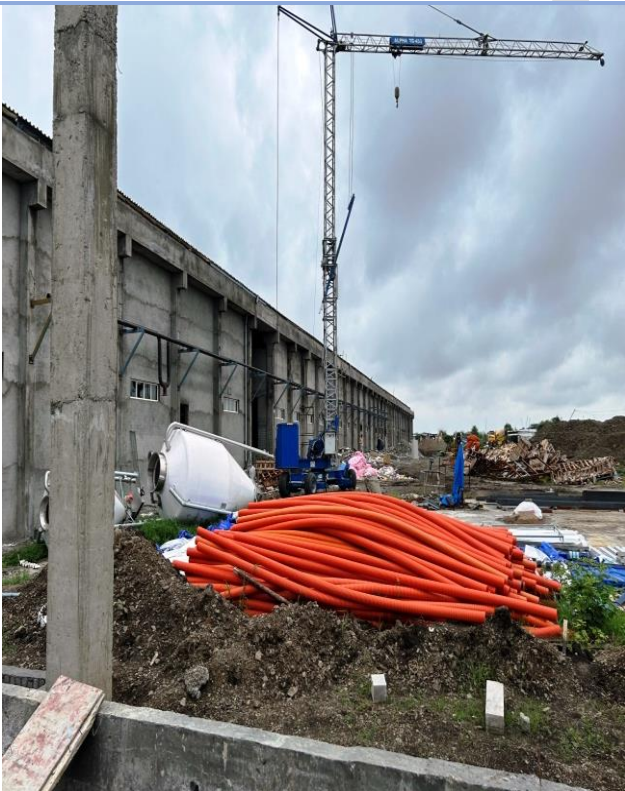
View of Warehouse-1 (Main Plant Building)
