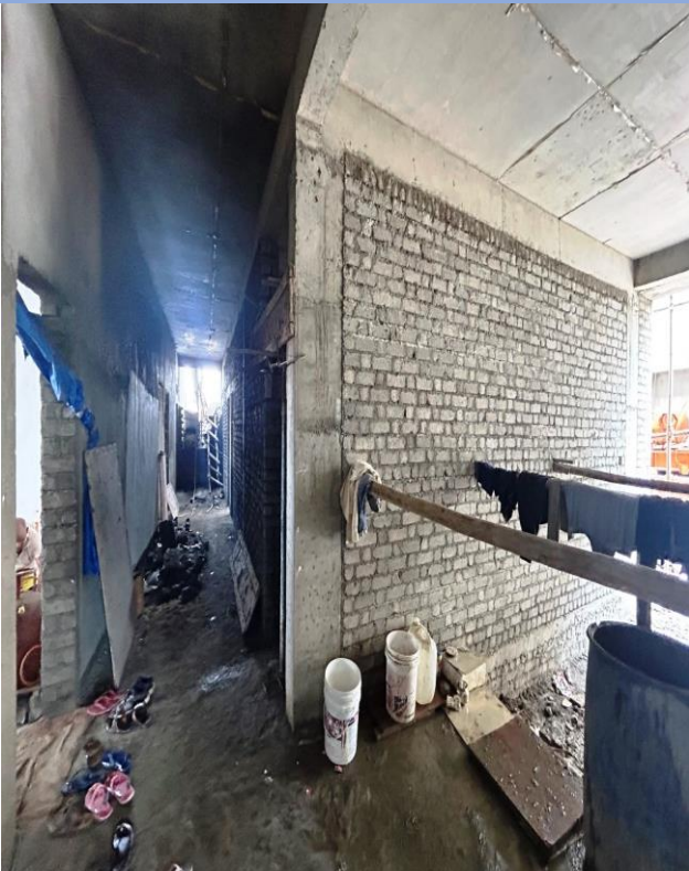
Internal View of Male Quarters
