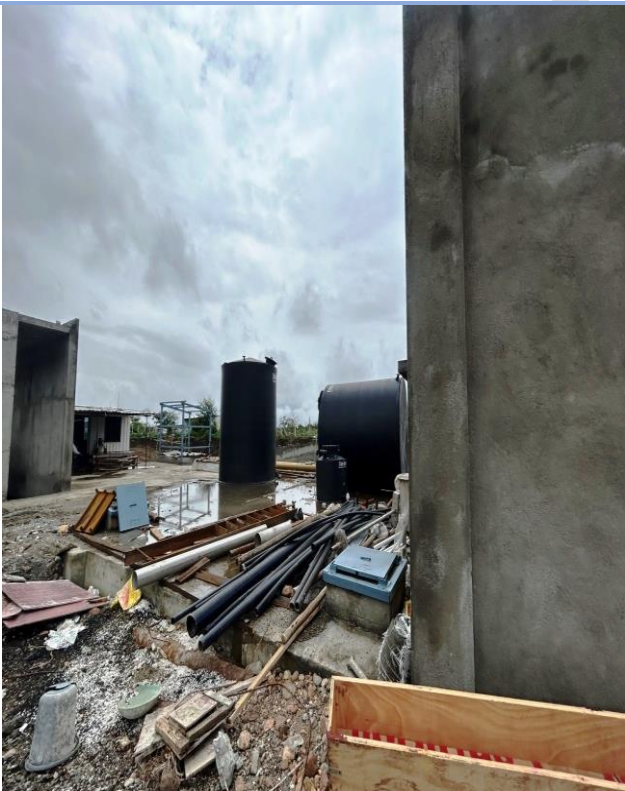
Under Ground Water Tank
