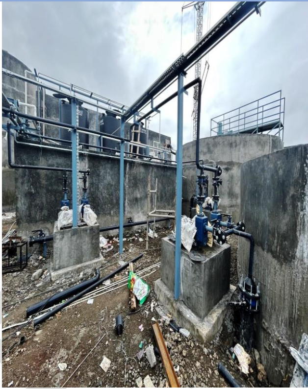
View of ETP
