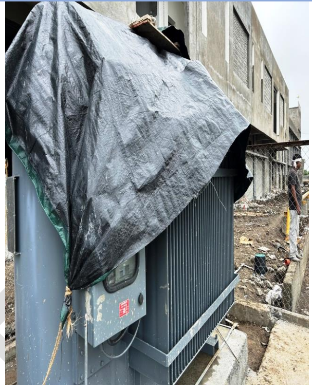
Hermetically Sealed Distribution Transformer-1600 KVA (OLTC Indoor), Sr. No. DI-31803
