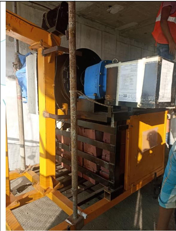
Floor Crane at Worli Site
