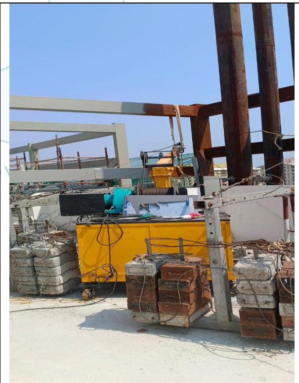
Floor Crane at Bagmane Bangalore Site
