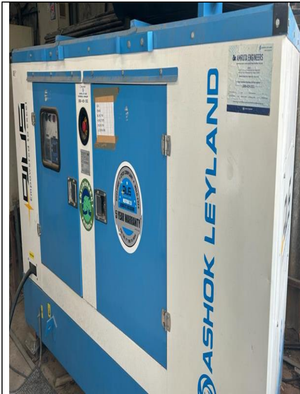
Diesel Generator-82.5 KVA at Bangalore Factory
