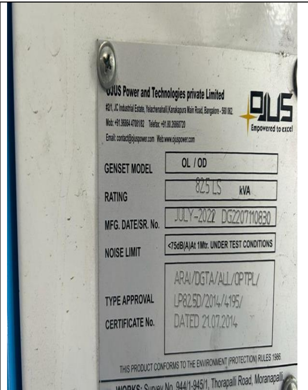
Diesel Generator-82.5 KVA at Bangalore Factory
