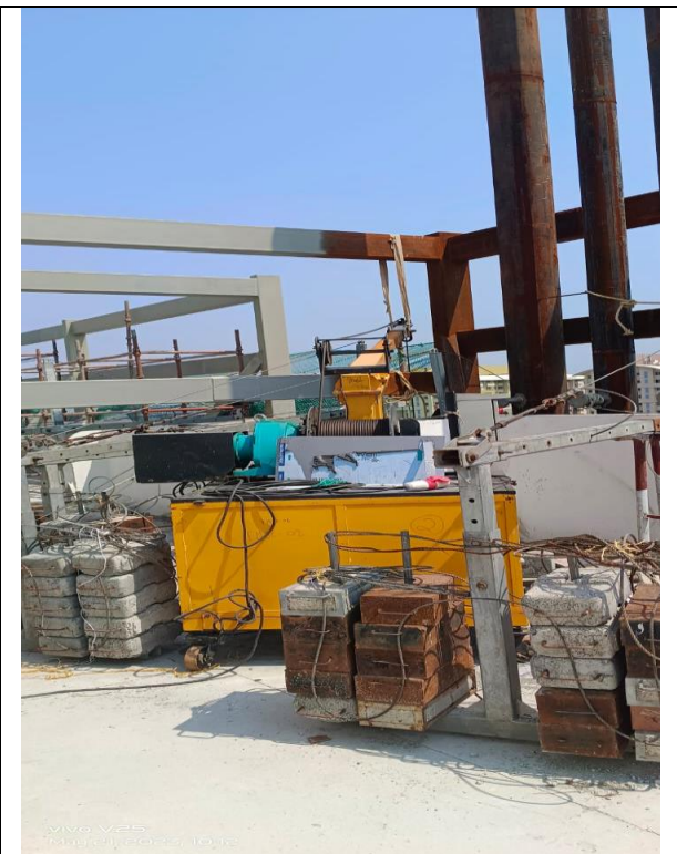
Floor Crane at Bagmane Bangalore Site
