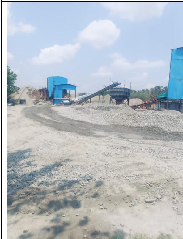
View of Stone Crusher Plant
