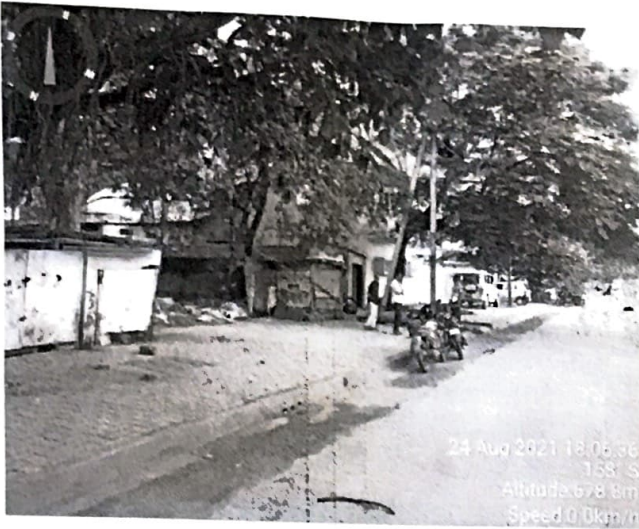
Side View With Approach Road
