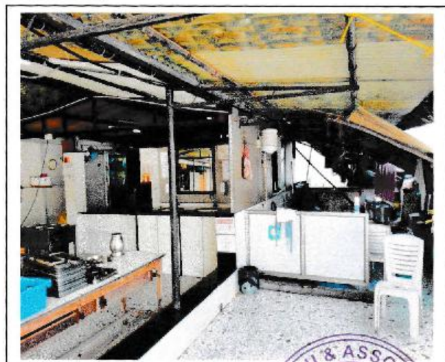
View of the Terrace Floor
